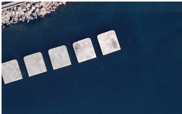
Figure 6.6: Breakwater structure in Sant Feliu de Guíxols. Image credit: Map data ©2017 Google.
